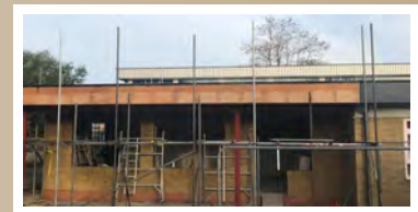
Photo: Scaffold being struck on an extension to Grays Convent School
