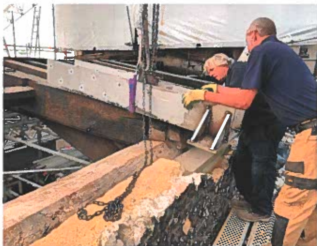
Installing new stainless steel flitch plates and brackets to extend the principal rafters across to the new outer wall plate
